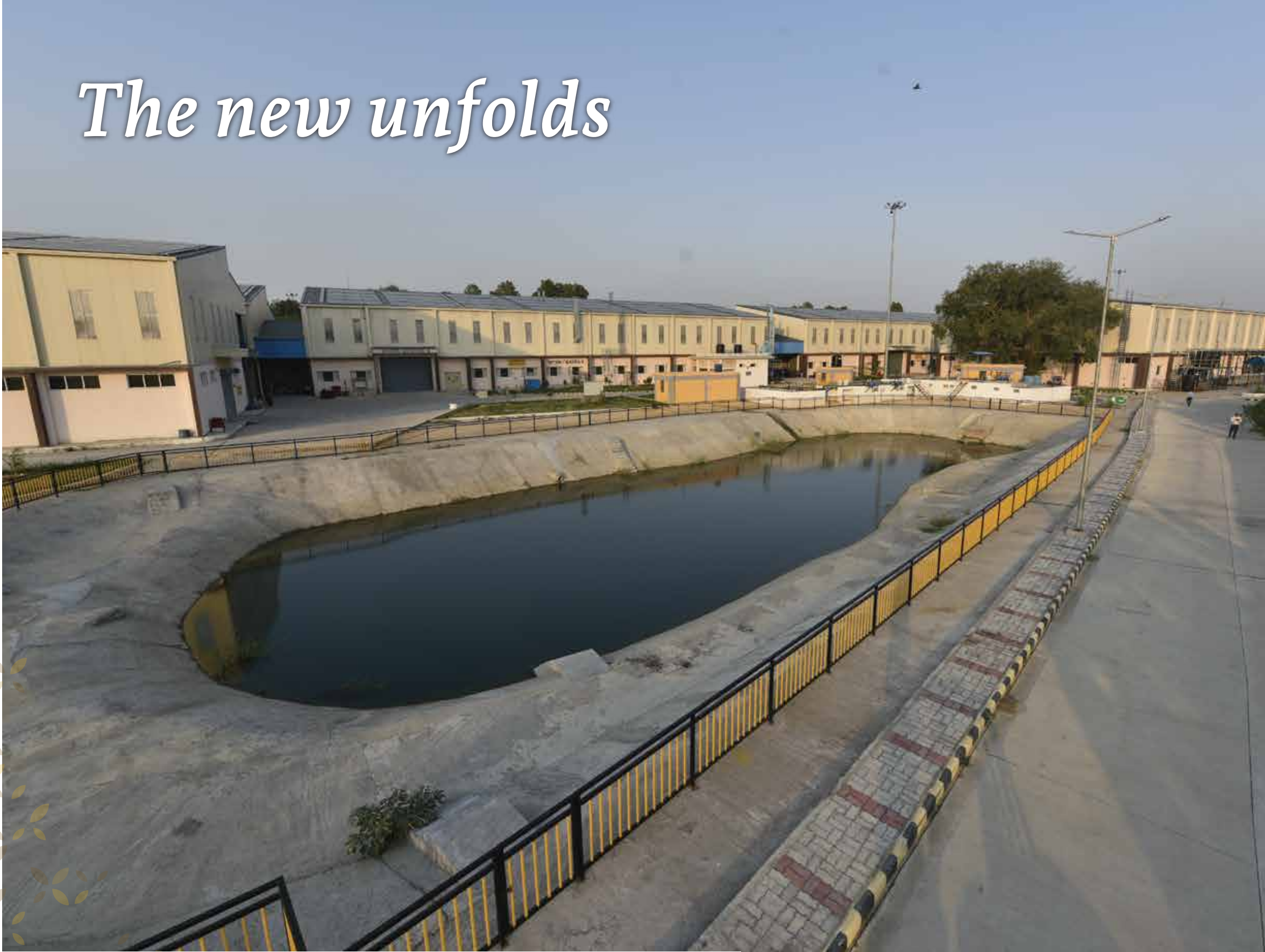
Wide angle view of the new workshops and pond as reservoir for treated water of ETP plant
